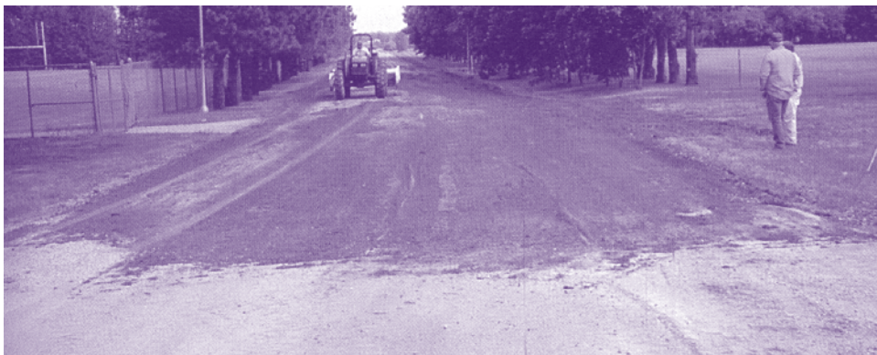
It is good practice to loosen, mix, and reshape gravel in a washboard prone area while it is moist.
