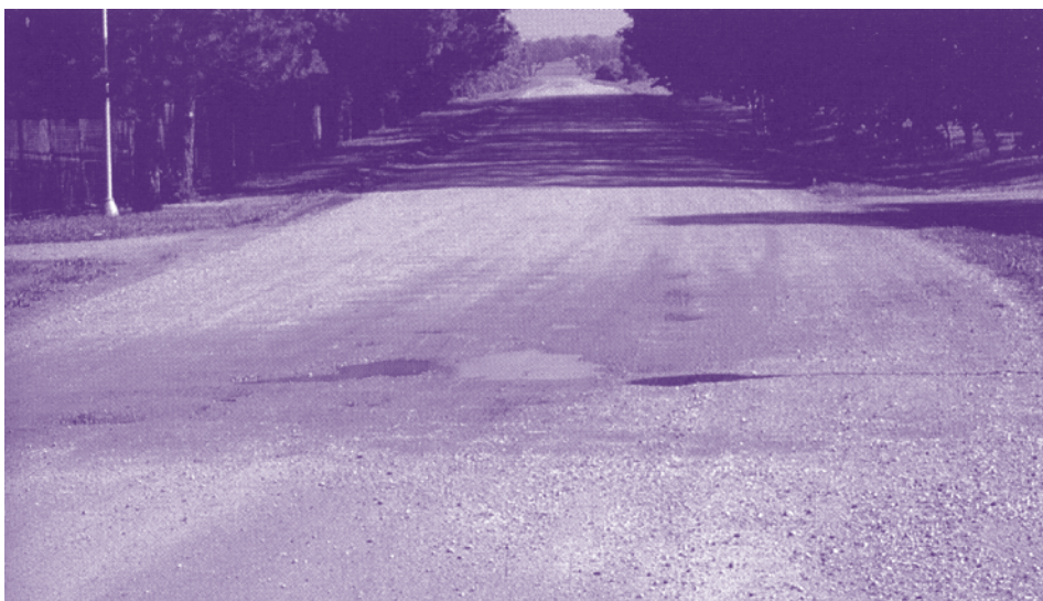
Another washboard-prone area is at the transition from paved to gravel sections as shown in this photo.
