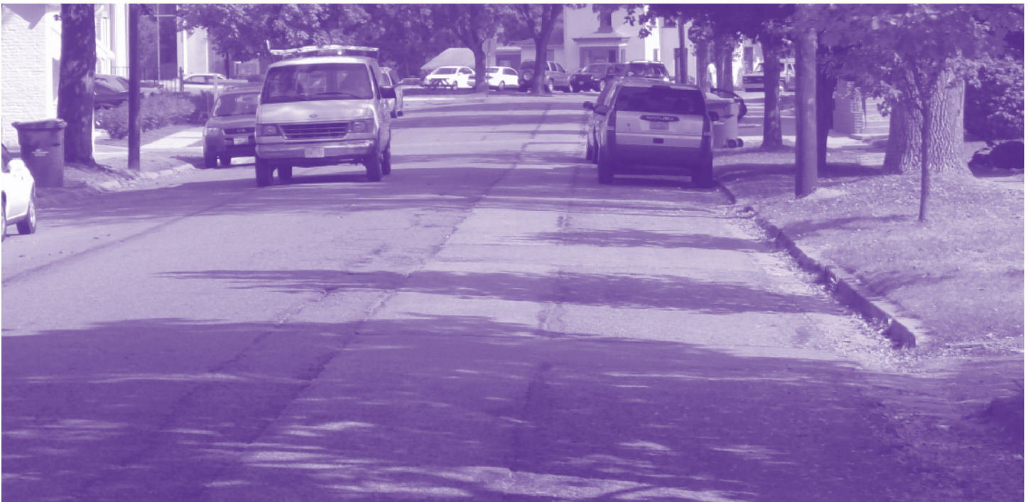
Before construction: Pavement, gutters and sidewalks were seriously deteriorated. (Photo: Stephen Farst, EMH&T, Inc.)
