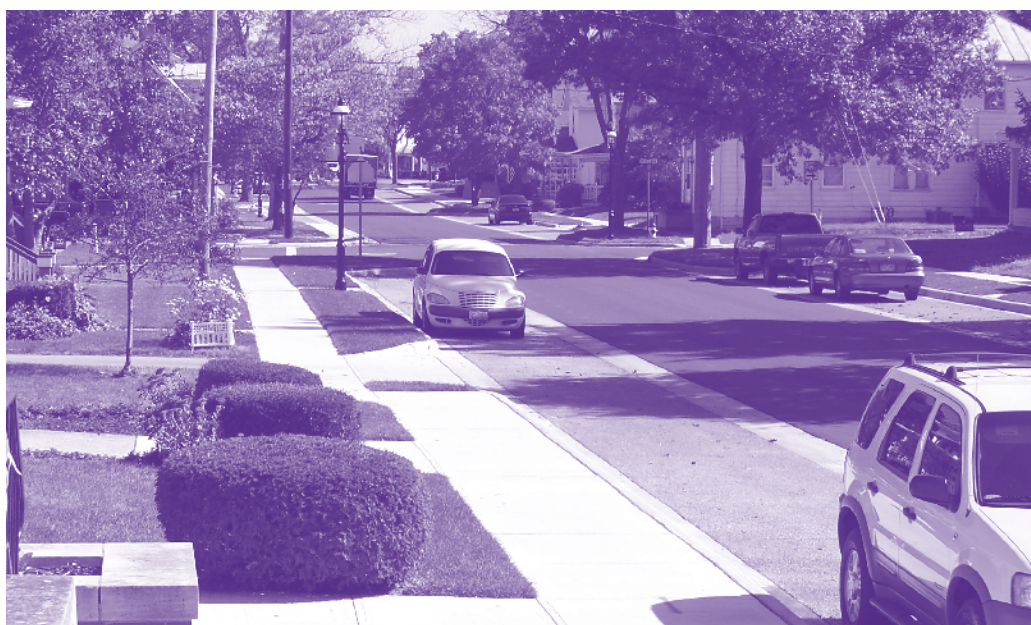
Finished street: Pervious paved parking bays integrate well into newly reconstructed travel lanes. (Photo: Stephen Farst, EMH&T, Inc.)
