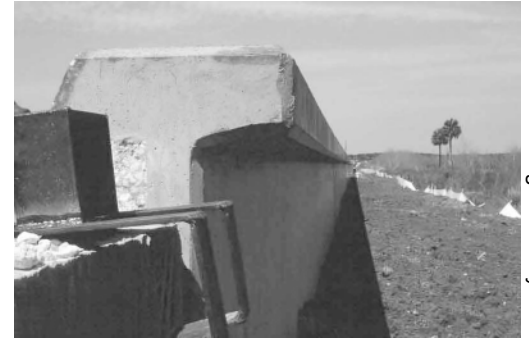
Profile of barrier wall during construction.
