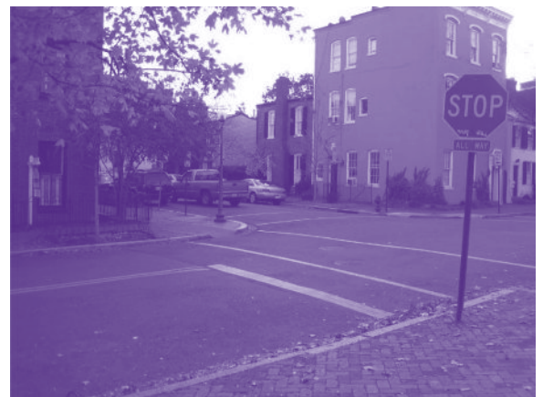
Figure 2: Enhanced Pavement markings (double-yellow centerlines and stop bar)
