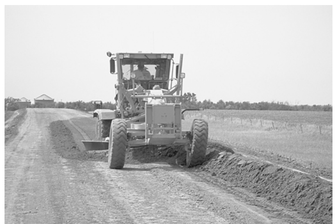
When reshape is finished, good quality surface gravel should be placed quickly before rain causes subgrade to lose its shape.
