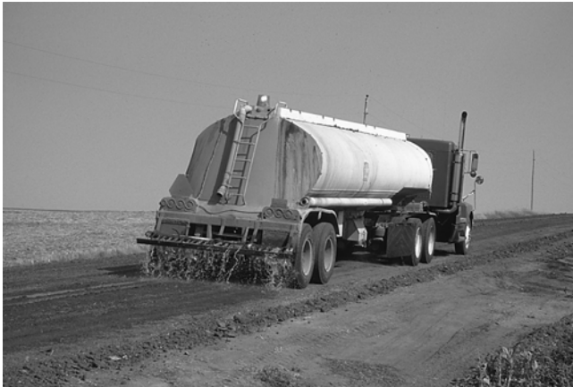
Reshaping can be done without these, but a water truck and rollers are very helpful tools to recompact material.
