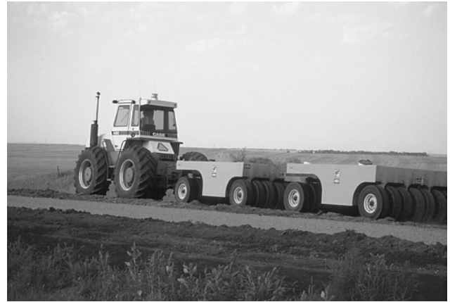
Reshaping can be done without these, but a water truck and rollers are very helpful tools to recompact material.
