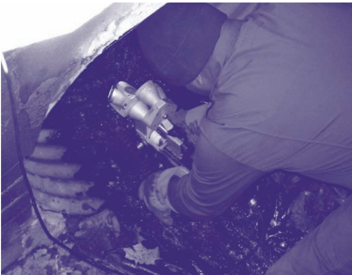
Willy Wilbur places the Rover ® in the culvert
