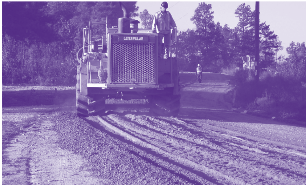
Mixing cement during the FDR process
