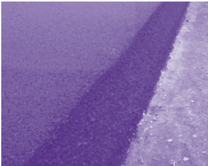
Illustrating the taper between the roadway pavement and graded shoulder. Photo courtesy of Gary Antonelli, President, Advant-Edge Paving.
