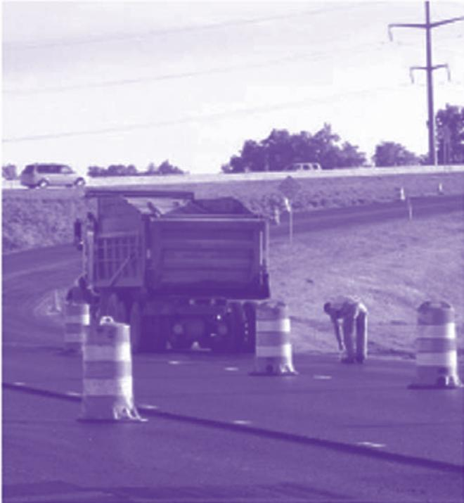
On July 18, 2006, a 21-year-old road construction worker was killed when a dump truck partially loaded with asphalt backed over him. The victim was working at night on a state highway paving project. The dump truck driver was backing through the work zone with the truck's back up alarm sounding.
