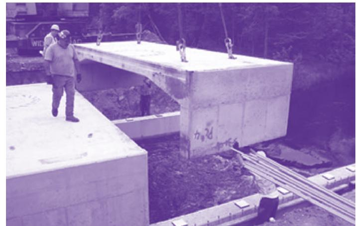
**The mid-section of the precast superstructure for a bridge on M-115 is placed as part of the Michigan Department of Transportation’s performance contracting project.**
