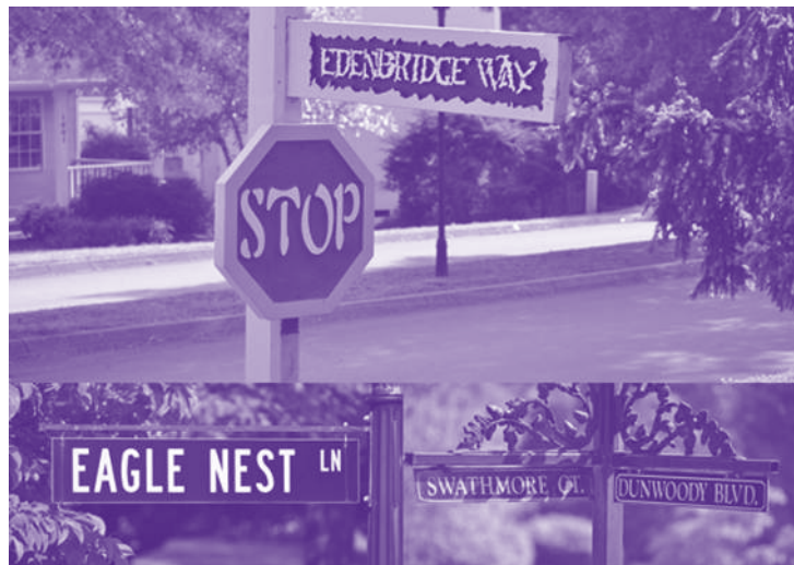
These ornamental street name signs fail to meet MUTCD requirements for color, legibility, letter height, and/or retroreflectivity. The top sign is almost illegible under perfect conditions and will provide little if any benefit during nighttime hours.
