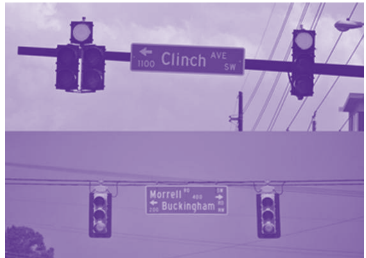
Overhead signs place street name information in a prominent location, particularly at signalized intersections. Also note the size of the lettering (12") relative to the adjacent signal indications.
